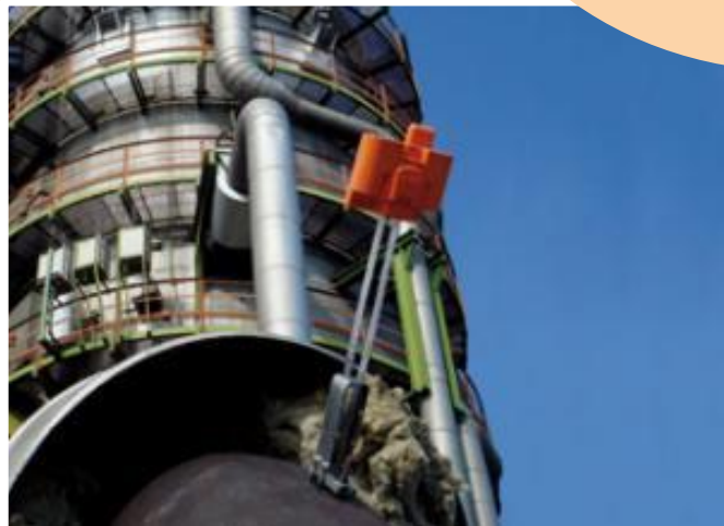
Insulation replaced after sensor mounting
