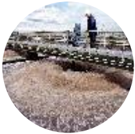
Industrial water treatment
