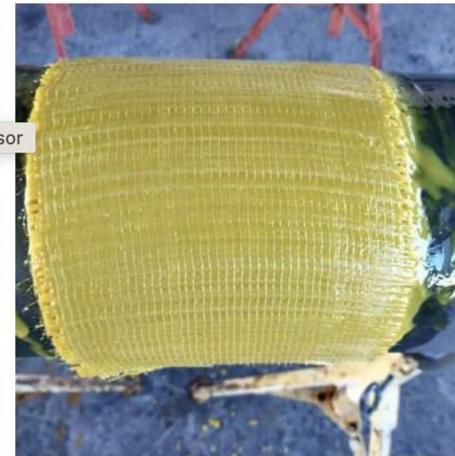
Composite repair applied over sensor.
