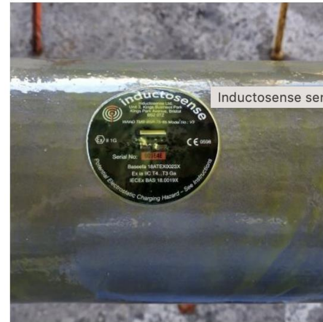
WAND TM Sensor installed on 6" pipe.
