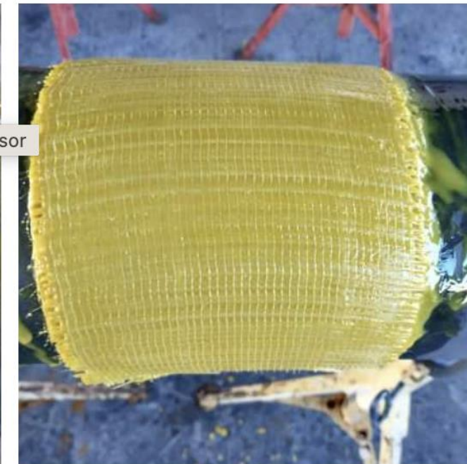
Composite repair applied over sensor.
