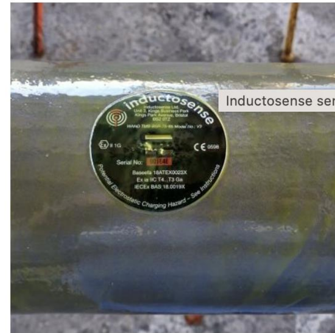
WAND TM Sensor installed on 6" pipe.
