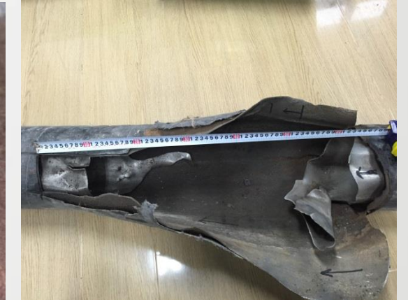
Clad Pipe Bursting
