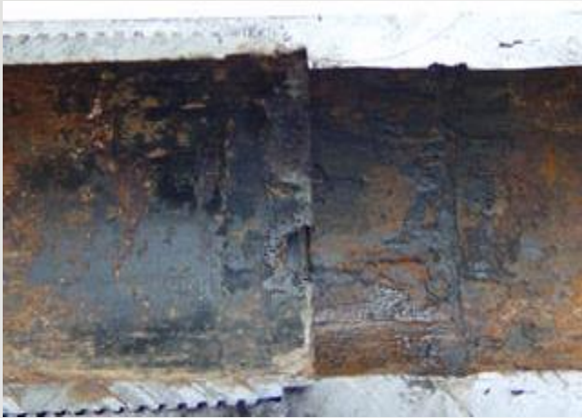
Tubing CO 2 Corrosion
